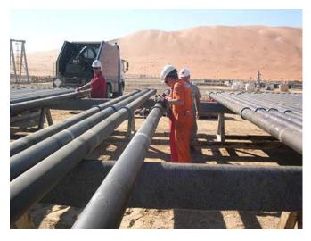
On Friday 13 July, a 5 1/2" x 17 lbs/ft VM50 VAM® ET WISE expandable string was successfully run (with no rejects) and expanded in the 7" section of a well in the Middle-East desert. The objective is to develop a weak producer. Deepening the existing horizontal hole, then sidetracking and drilling an additional two laterals. This will maximize the reservoir contact and improve the productivity.
